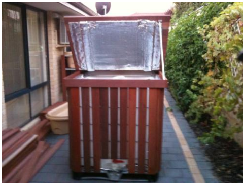
Figure 3 Tank with Jarrah wood decking screwed onto frame and insulated lid attached. Note that the insulation was stapled to the wood to block light and heat from the tank except for the front of the tank, to allow some light in for fish health
