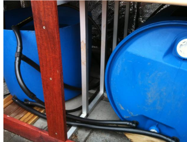
Figure 6 The sump system uses one full and one half blue barrel on each side. The water pump, a 2400 Litre per hour 35 watt submersible pond pump, pumps water three places - into the upper growbed, the lower growbed, and the fish tank
